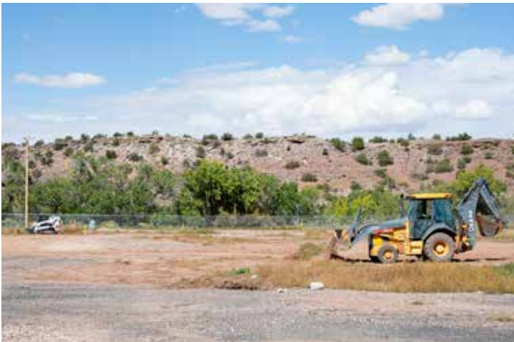
Photo - Facility Department preparing area for the project.
